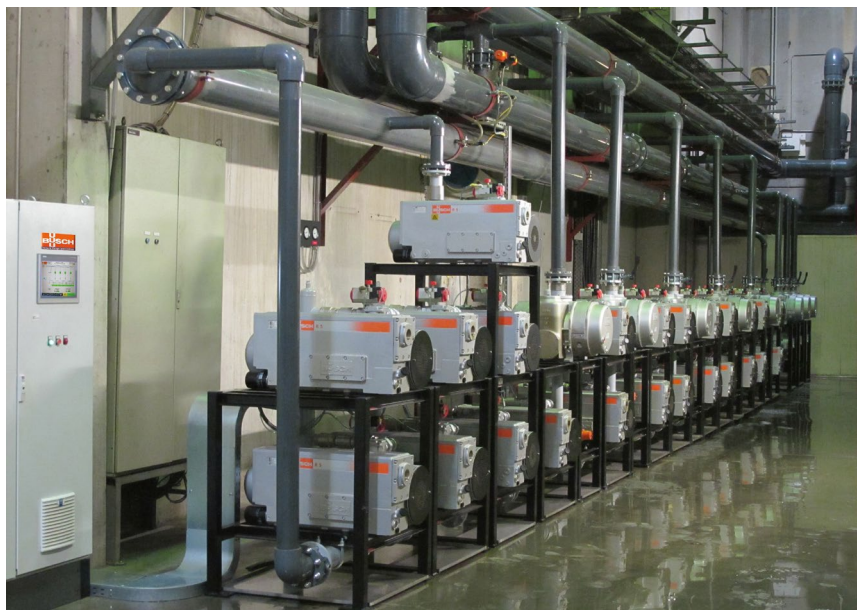
Figure 14 Example of a fully centralized vacuum supply
